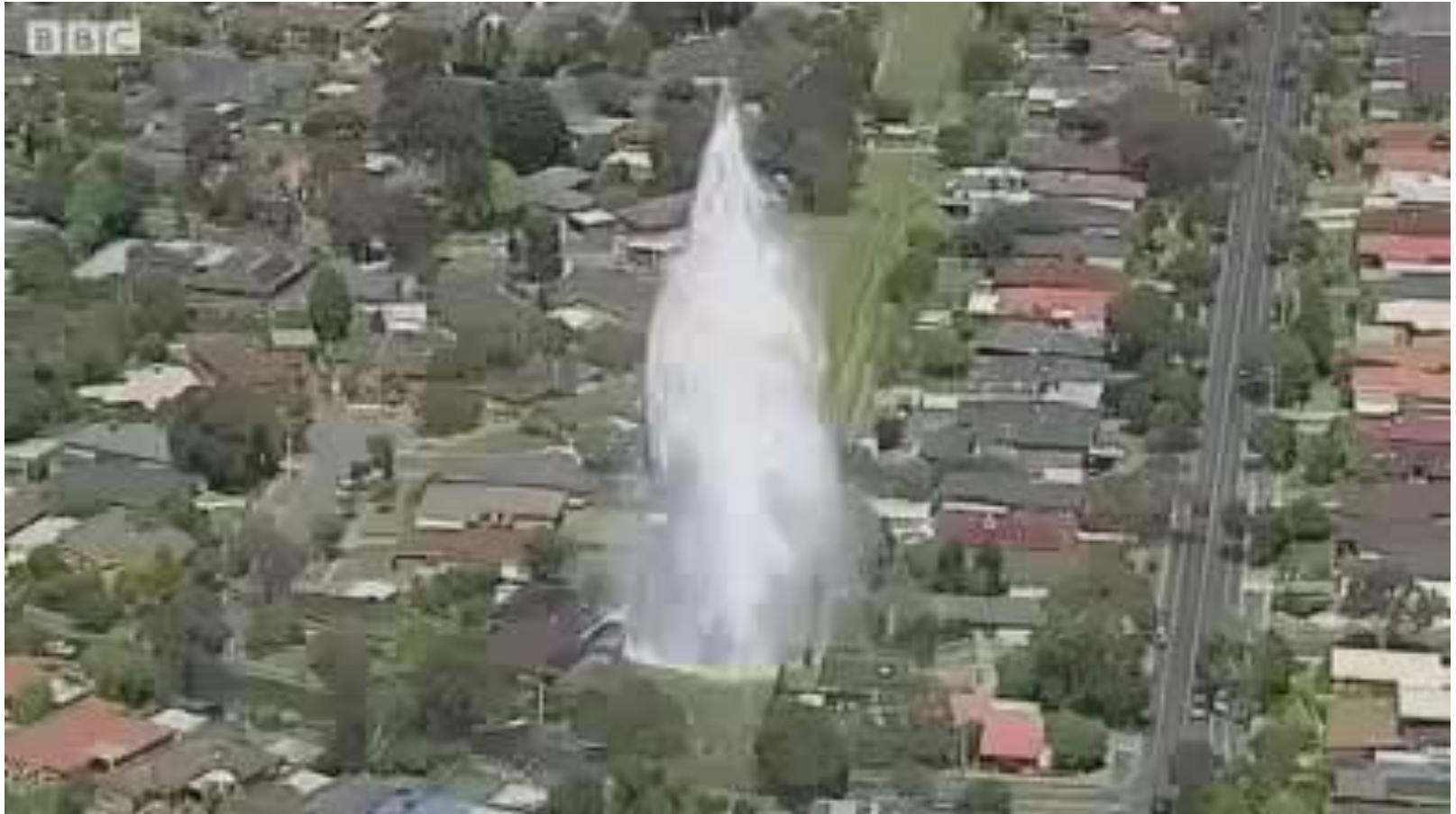
Burst water main: Australia
