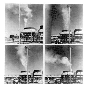
Figure 10. Recirculation in Induced Draft Air Cooler.
